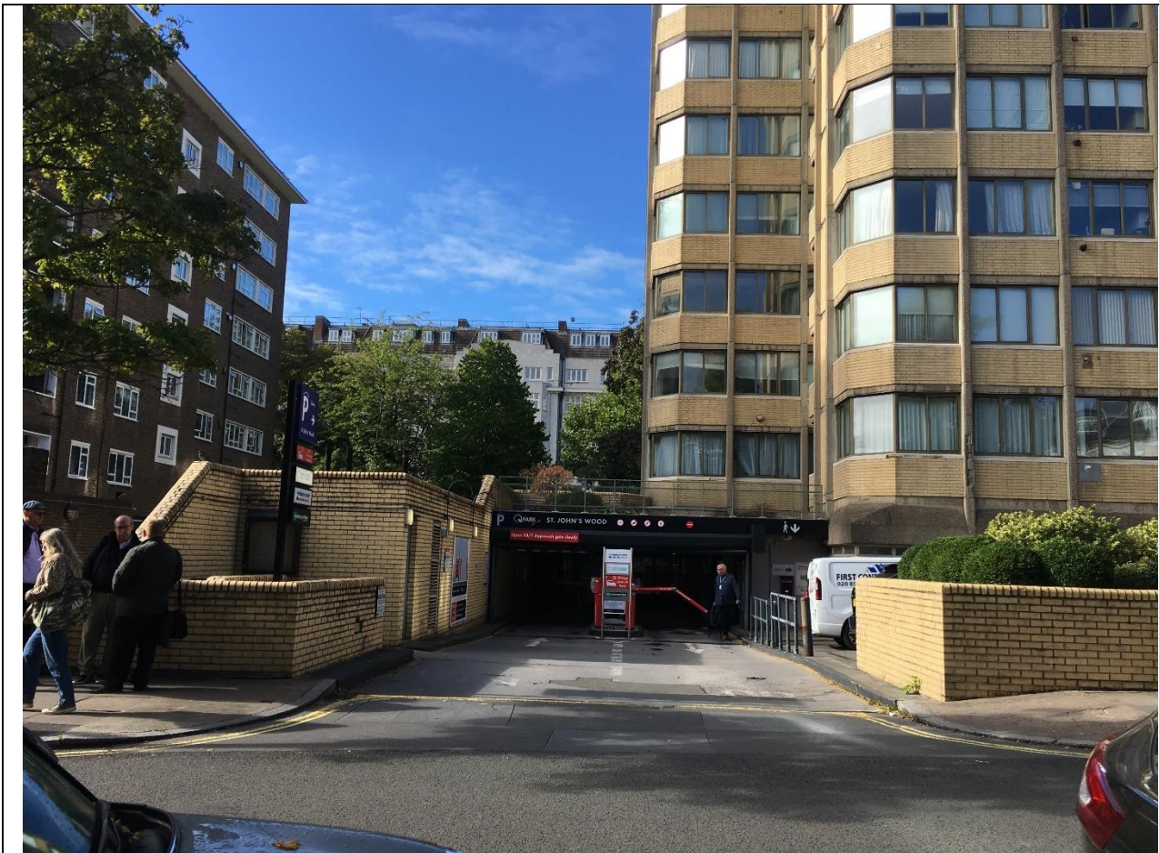
Kingsmill Terrace – Vehicular & Pedestrian Access to Public Car Park and other commercial activities, sited below Birley Lodge, which is a residential development comprising three linked towers.
