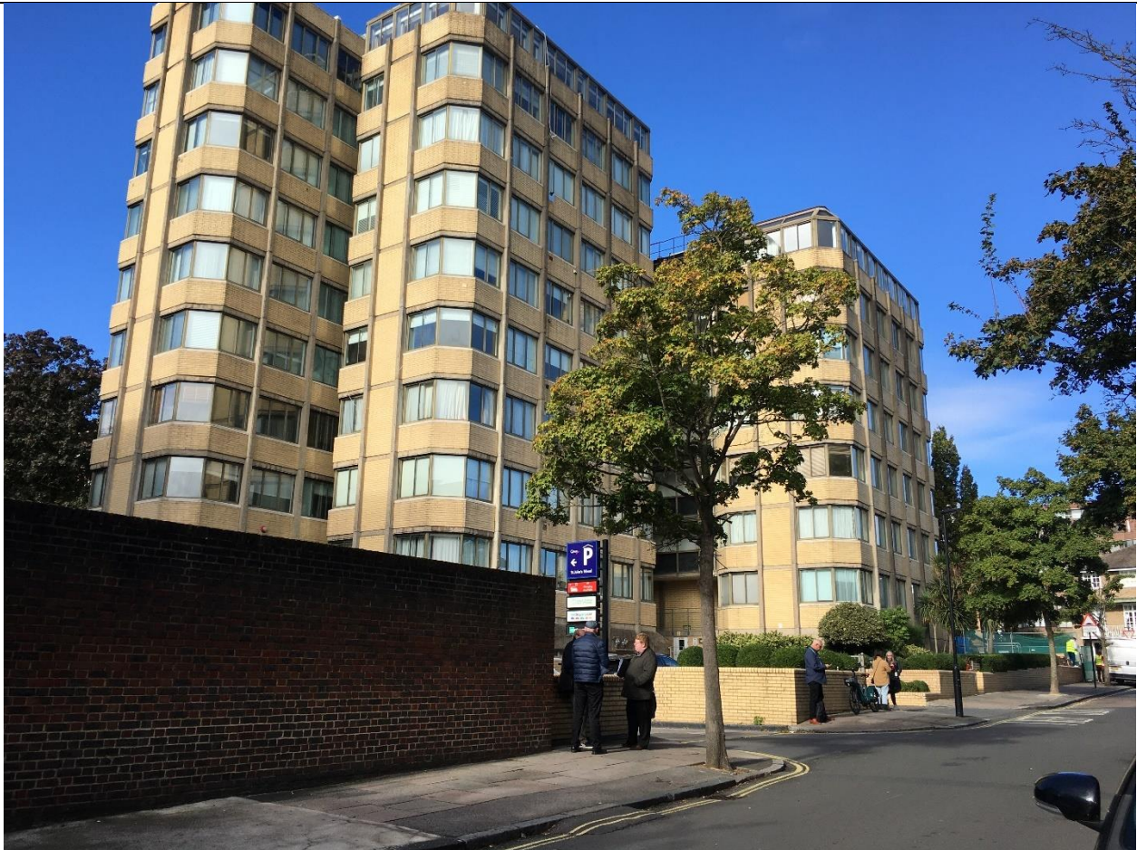
Kingsmill Terrace – Vehicular & Pedestrian Access to Public Car Park and other commercial activities, sited below Birley Lodge, which is a residential development comprising three linked towers.
